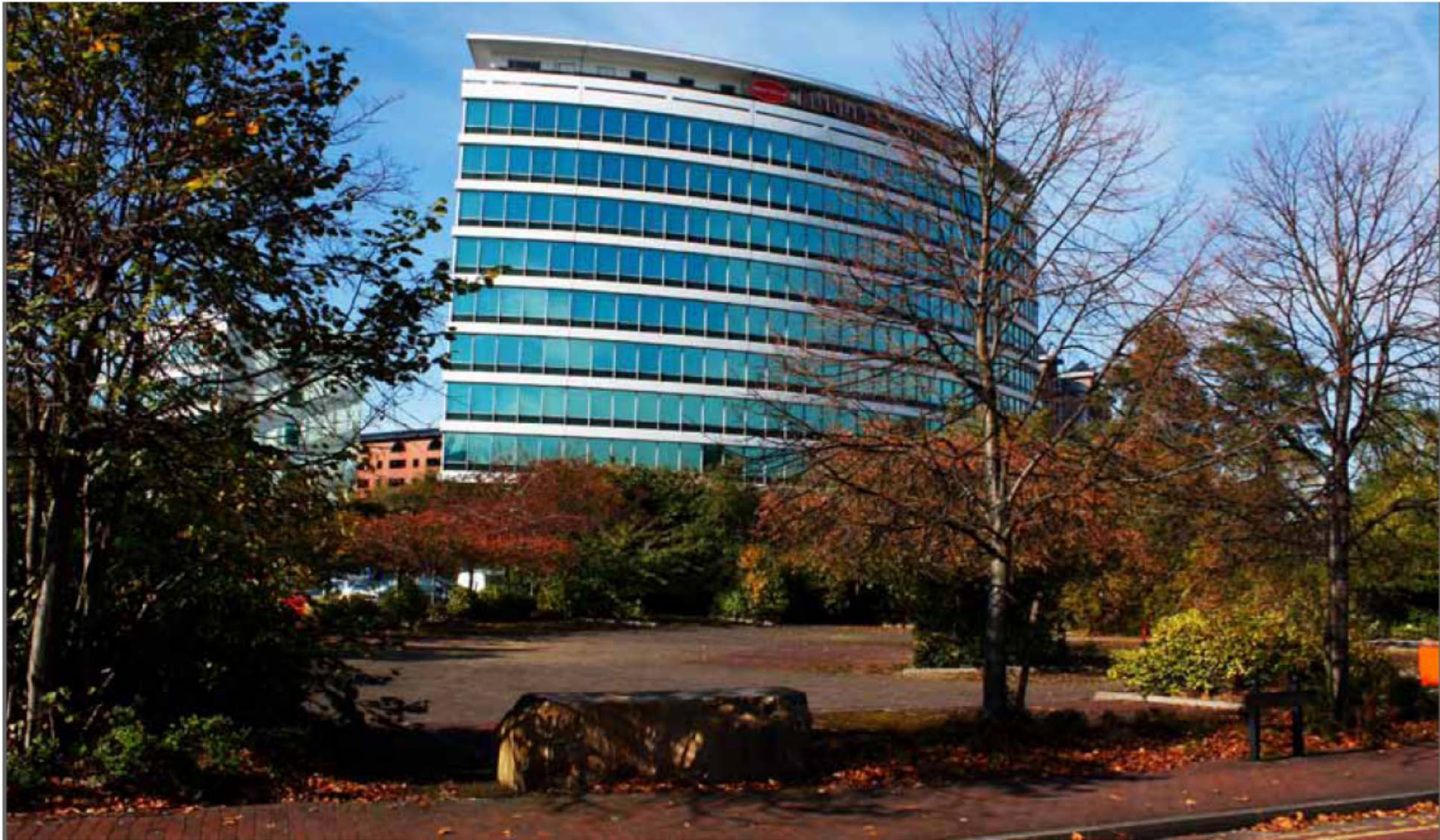
Salford Quays, Salford. Good planning ensures space to deliver a wide range of the benefits of green infrastructure alongside space for business. Picture by Martin Moss.
